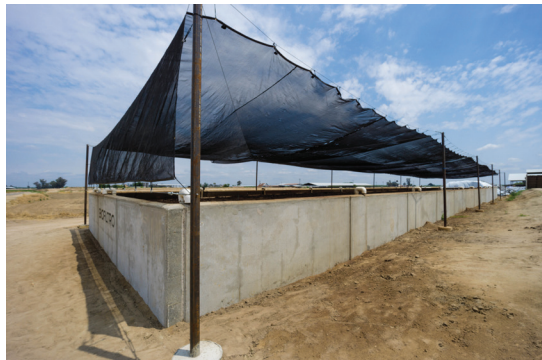
Side view of the BioFiltro system.
