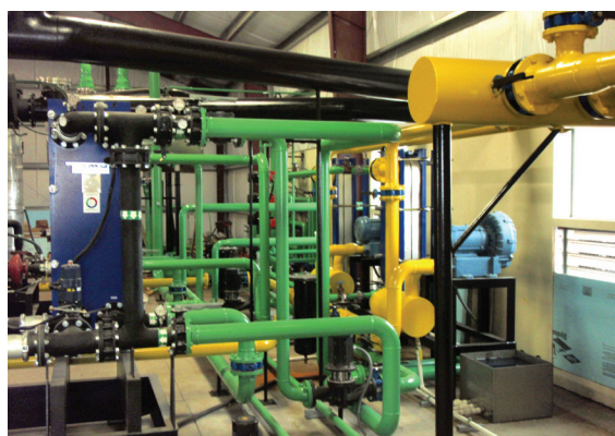
Gas, hot water, and gas recirculation mixing piping within engine/electrical building.
