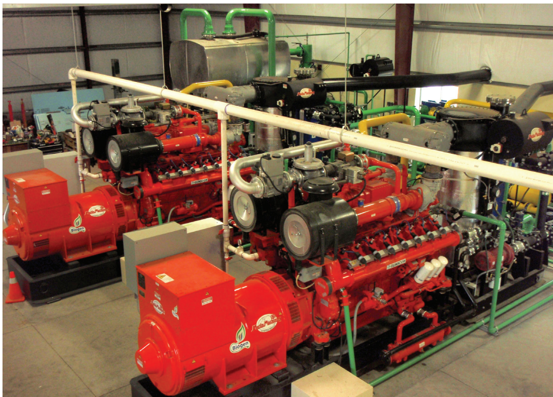
Two SFGD 560 Guasco engine/generator sets rated at 710 KW each.
