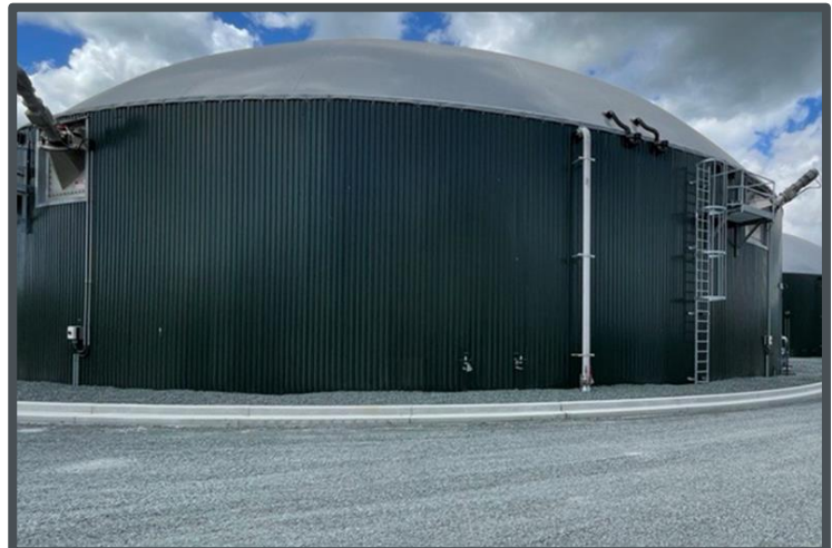
Figure 4: Digester Tanks
