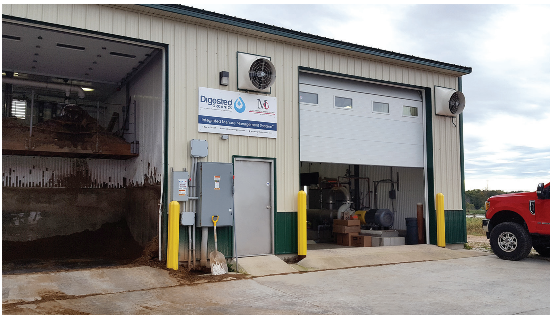
Digested Organics NCWRS screw presses, fiber storage and UF, Majestic Crossing Dairy
