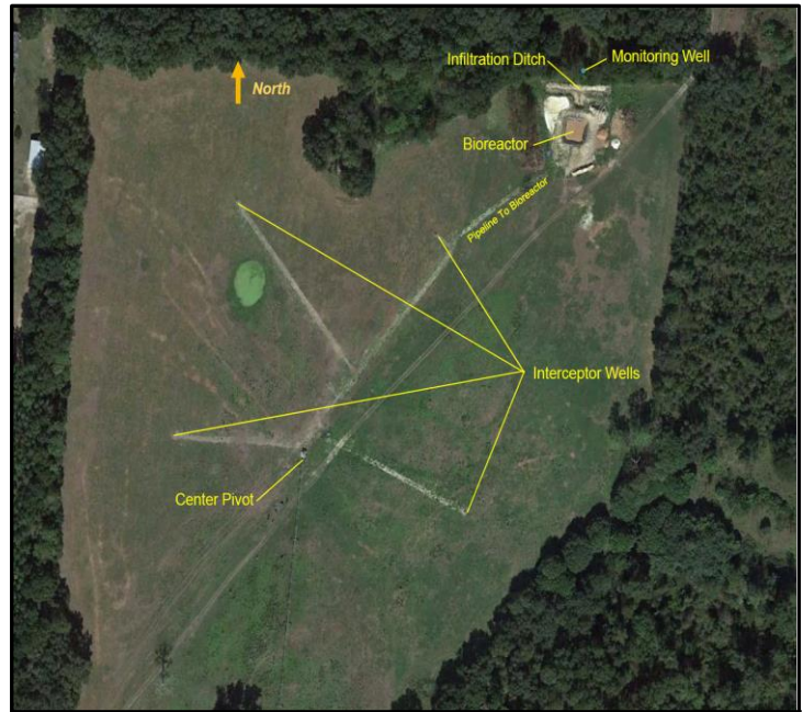
Figure 3. Watson Interceptor Wells and Bioreactor
