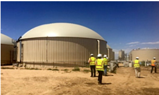
Figure 5. Six complete mix digesters - 1.7 million gallons each.
