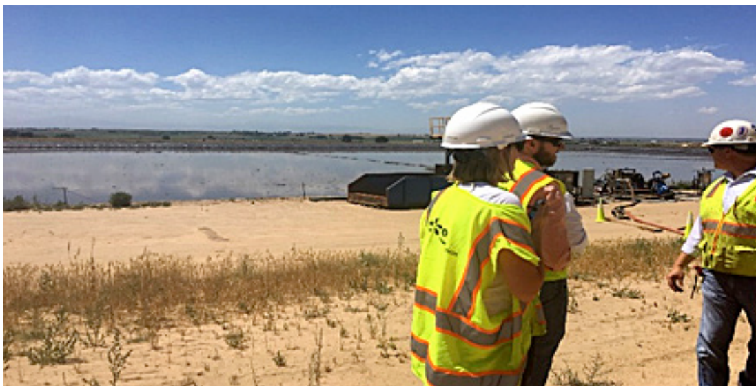
Figure 8. One of two liquid byproducts holding ponds. Total on-site capacity 42.8 M gallons.
