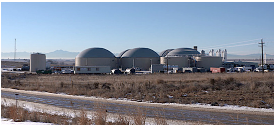
Figure 1. Heartland Biogas Project – Weld County, Colorado.
