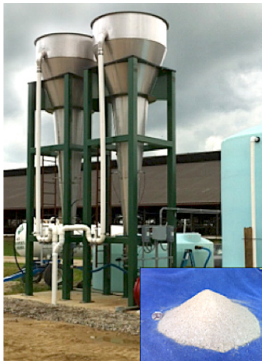
MultiForm Harvest Struvite Crystallizer Jones Family Dairy, Massey, MD
