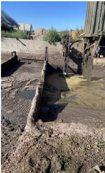
Figure 1. Sand separation unit in Hood Family Dairy
