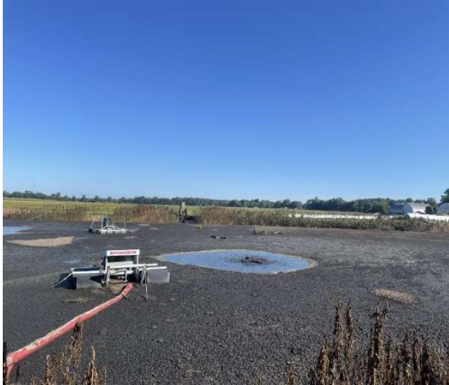
Figure 2. Pond with aerators installed.
