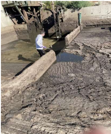
Figure 6. Sampling from inflow stream located at the exit of sand separation.
