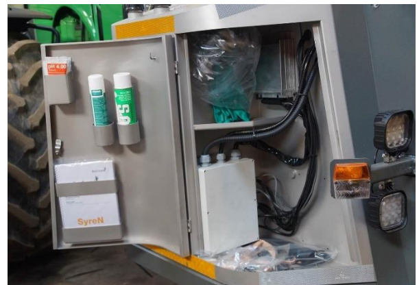
Figure Side cabinet on SyreN with electronics and safety equipment
