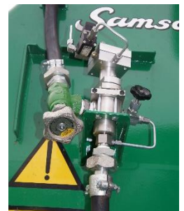
Ammonia injection valves
