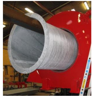
installing sleeve for protection of pressure tank
