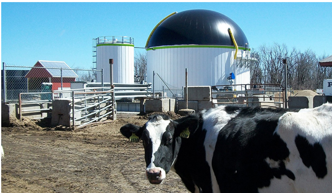
Anaerobic Digester at Jordan Dairy Farm.
